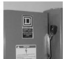
Figure 9-1 Power switch for machines with coolant-through-the-spindle option.
